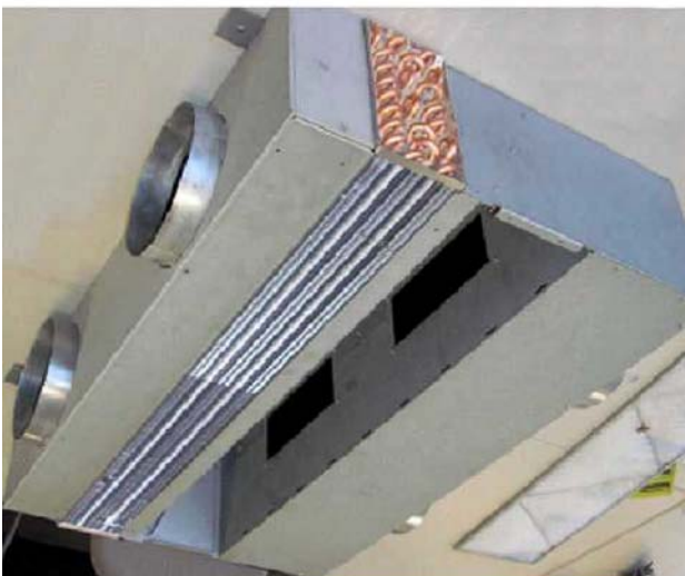
3. Removal of lower plate / vacuum-cleaning of heat exchanger on the pressure side
