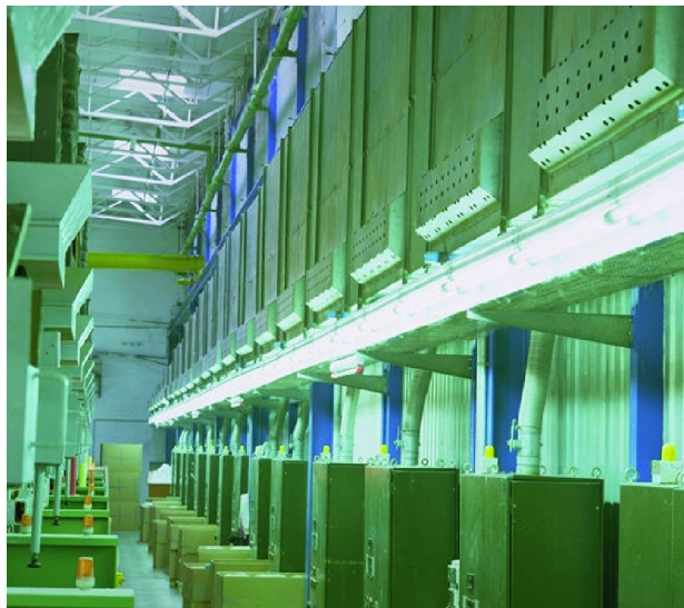
Air diffusers type LTB directly connected to the supply air duct, with lateral air injection.
