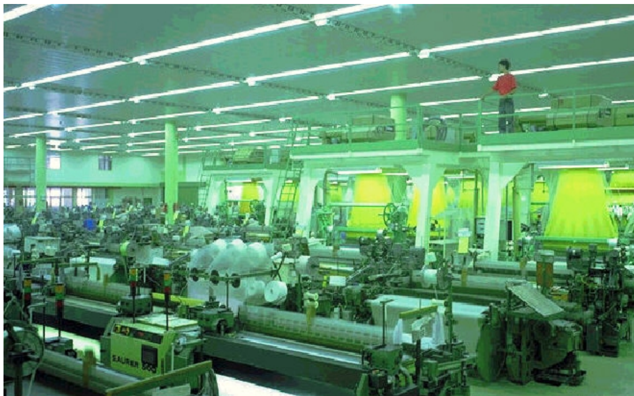
Air diffusers type LTB installed below the dropped ceiling with the supply air ducts above
