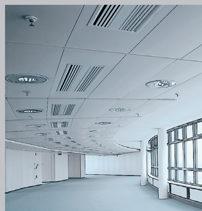
Example of usage: Foyer
